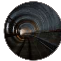
Drainage mats for tunnel construction
